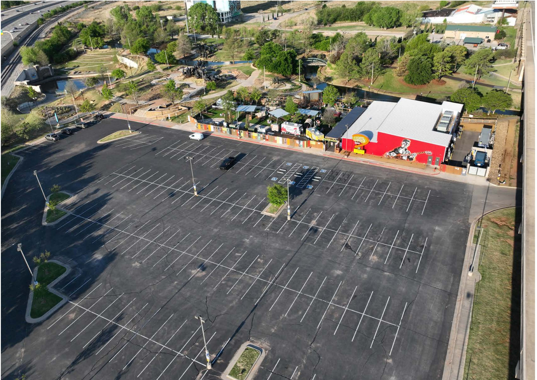
Existing driveway and parking lot in front of Truck Yard
