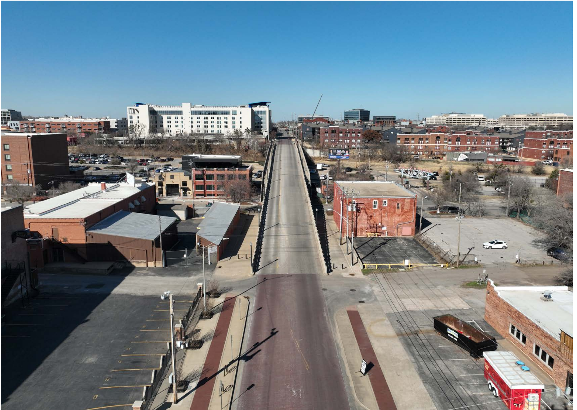
Existing Walnut Avenue looking North towards the bridge
